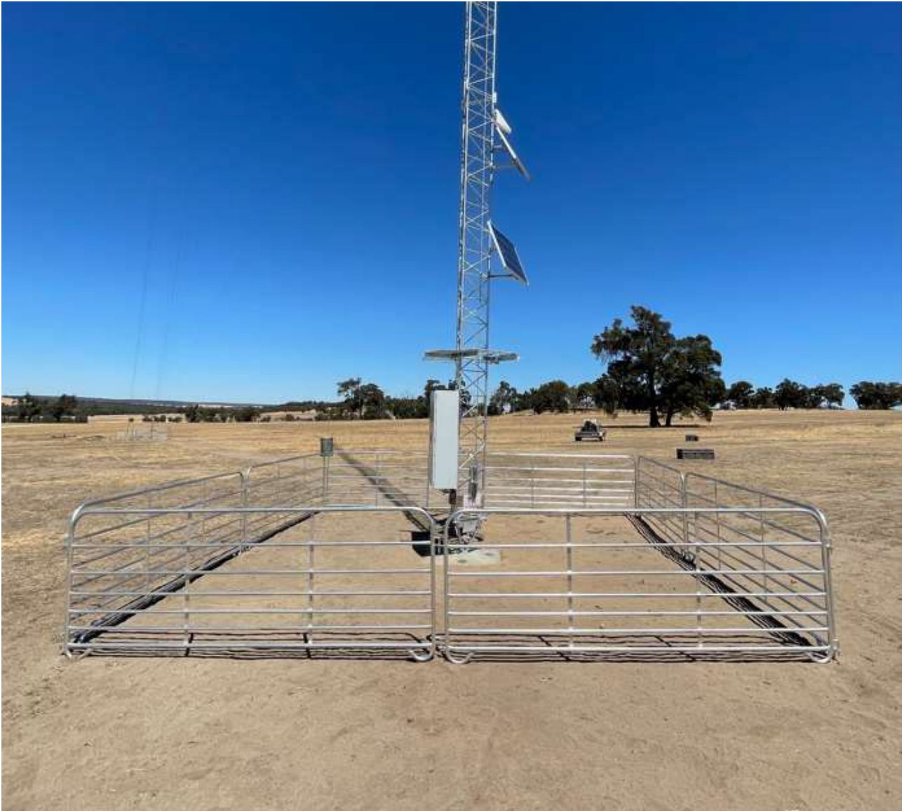
Plate 1.2 Met Mast base located in Shire of Narrogin
