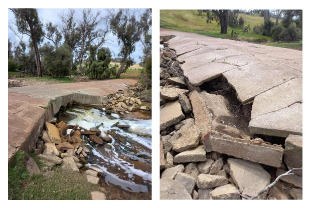
A quote has been obtained to replace the existing ageing culvert with a 750mm pipe, 9.6m wide with precast headwalls. Included in the quote is a new concrete deck to match the existing approaches. The total cost of the work, which includes the above-mentioned components, along with removal of in-situ material, is estimated to cost \$15,000.
