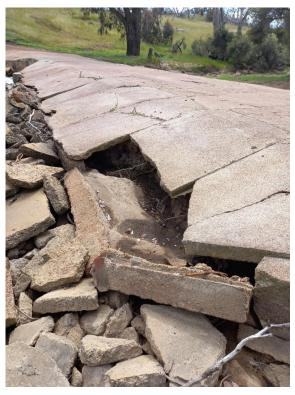
A quote has been obtained to replace the existing ageing culvert with a 750mm pipe, 9.6m wide with precast headwalls. Included in the quote is a new concrete deck to match the existing approaches. The total cost of the work, which includes the above-mentioned components, along with removal of in-situ material, is estimated to cost \$15,000.
