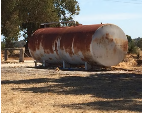
Photograph A: Onsite Whey Storage Tank
