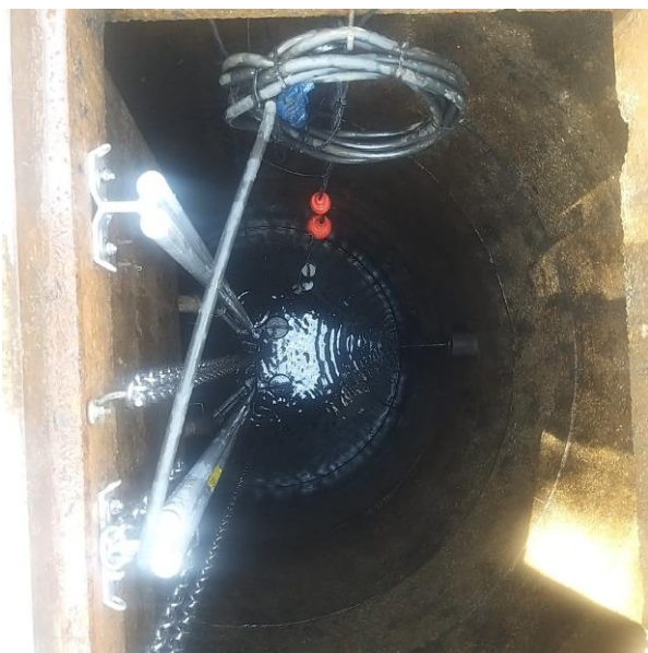
Pit re-build with new guide rails
