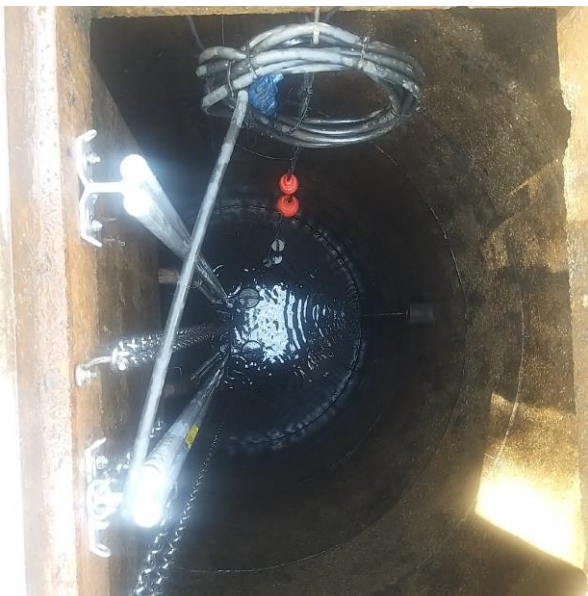
Pit re-build with new guide rails
