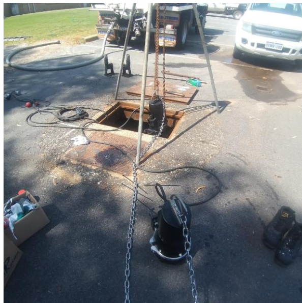
Pump installation and new chains
