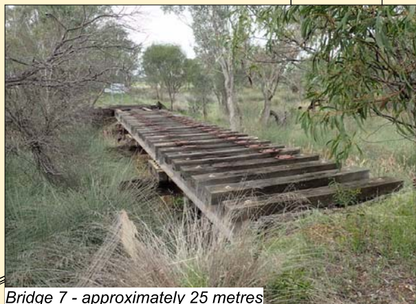
Bridge 7 - approximately 25 metres
