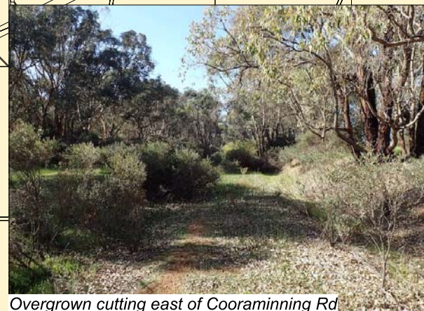
Overgrown cutting east of Cooramining Rd
