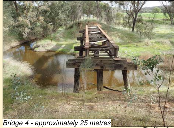
Bridge 4 - approximately 25 metres
