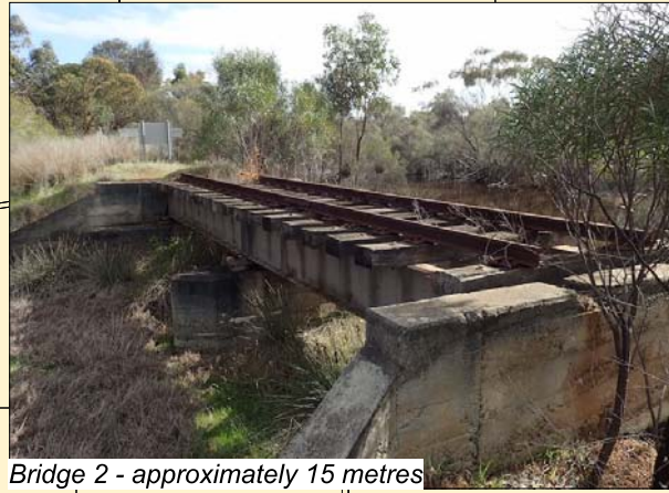
Bridge 2 - approximately 15 metres
