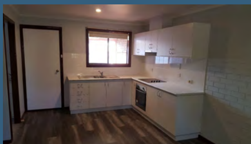
New Street Unit Refurbishment
