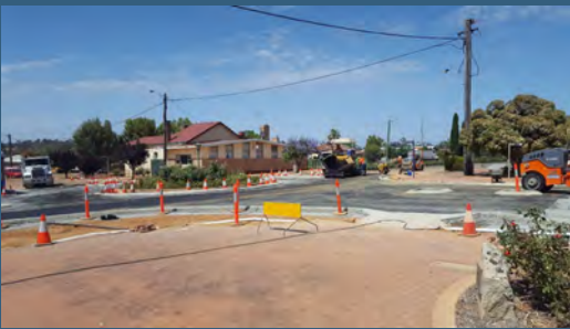
Asphalt installation on Brooking Street
