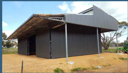
Williams Men's Shed Headquarters Under Construction
